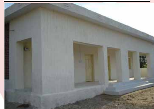
Front View of School
